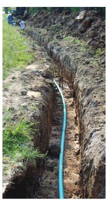
Small pressure sewer mains require only small trenches during installation.
