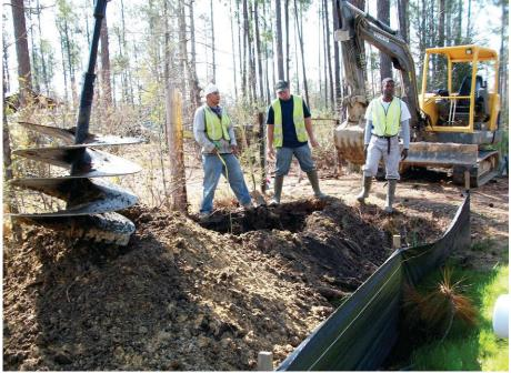
Use of a power auger is an efficient, clean, low impact method for installing E/One grinder pump tanks in the ground—site conditions permitting (photo credit: Compton Engineering, Inc.).
