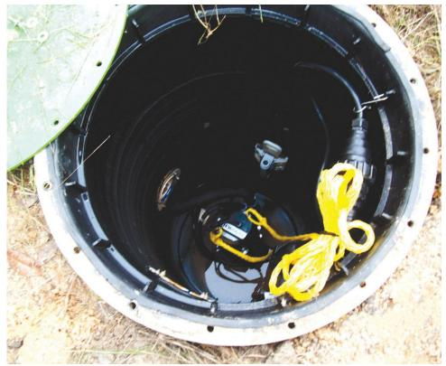
Top view of E/One grinder pump station.
