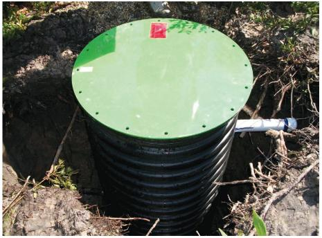
A high flood grinder pump station, rated for up to 15 feet of flood over cover, protects the integrity of the grinder pump system in flood prone areas (photo credit: Compton Engineering, Inc.)
