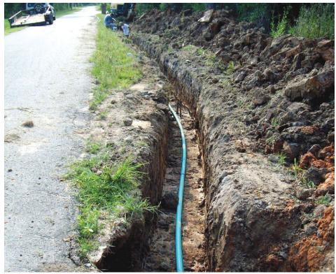
Small diameter flexible pipe being installed alongside roadway with minimum environmental disruption (photo credit: Compton Engineering, Inc.).
