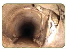
Gravity sewer main in need of repair.
