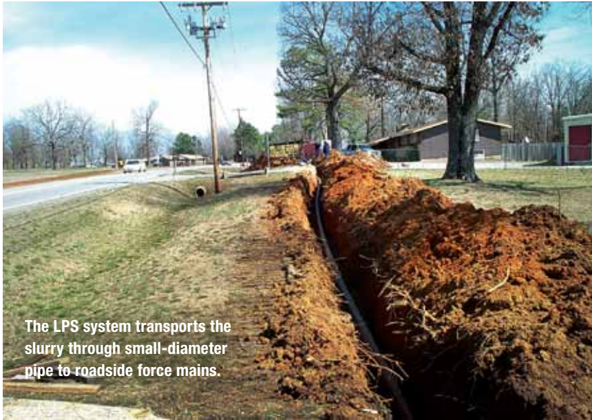
PHOTO COURTESY OF CRIST ENGINEERS INC.
